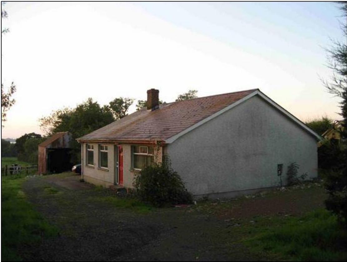
Plate 3 Bungalow close to eastern entrance of existing site
