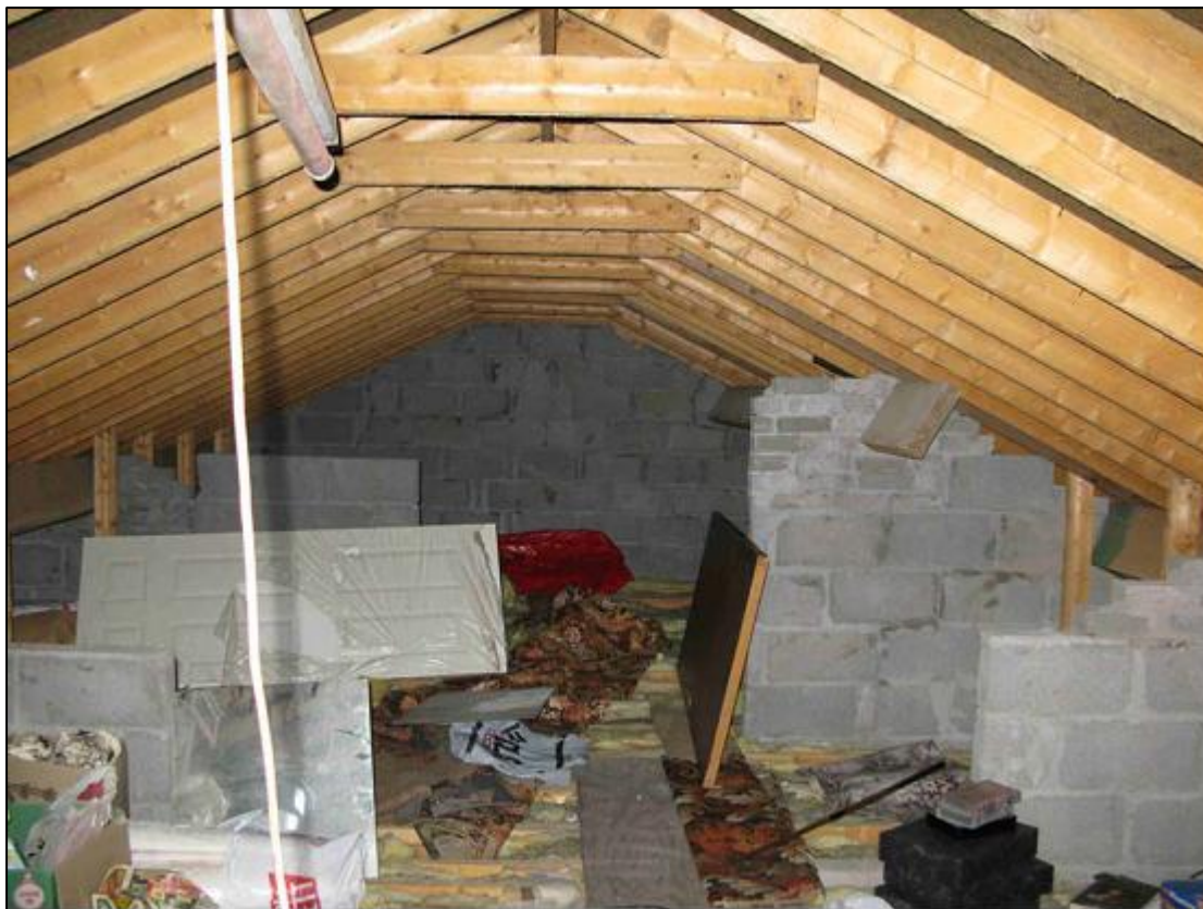
Plate 4 Roof void of the bungalow
